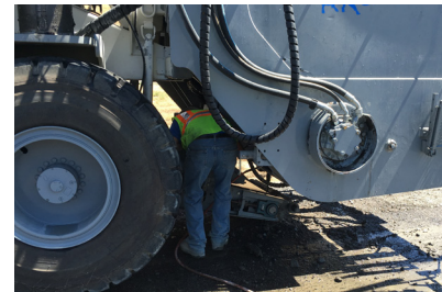
Jacking Columns and Hydraulic Lowering of Transfer Belt
